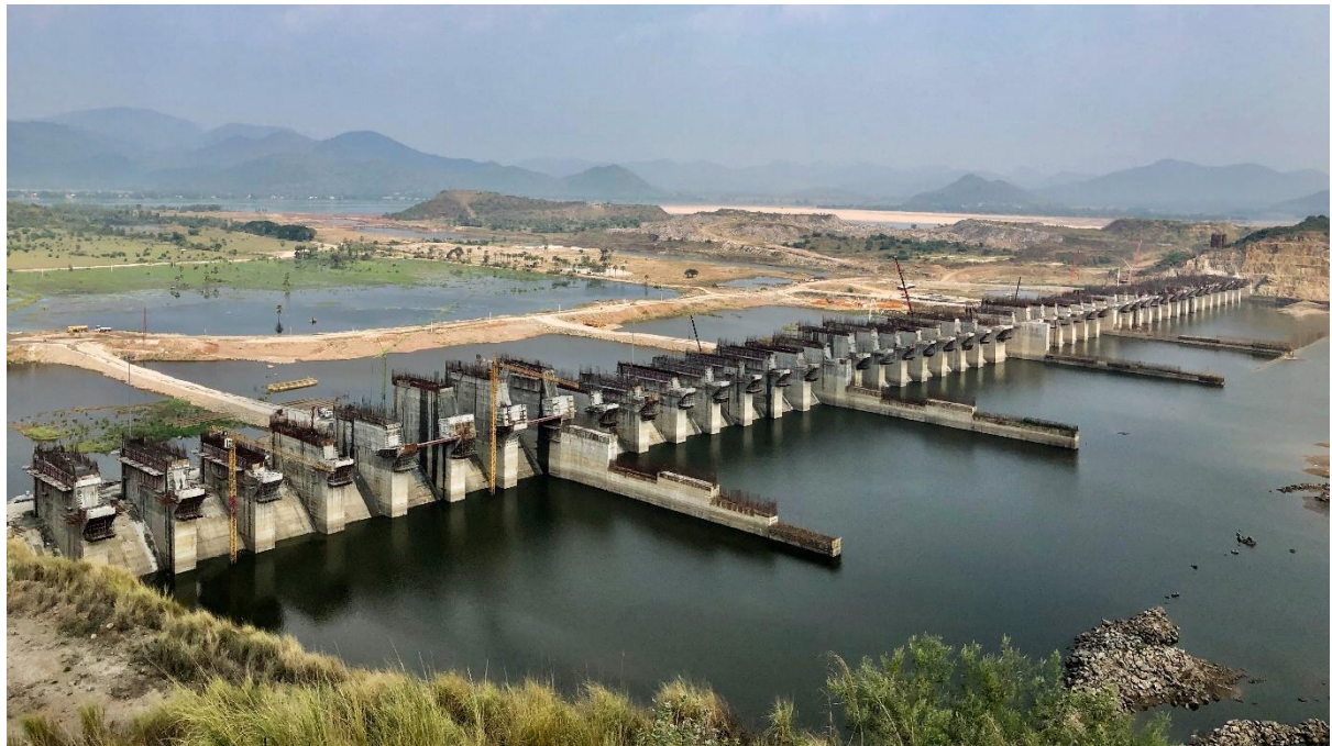
CONSTRUCTION SITE VIEW OF POLAVARAM PROJECT.
