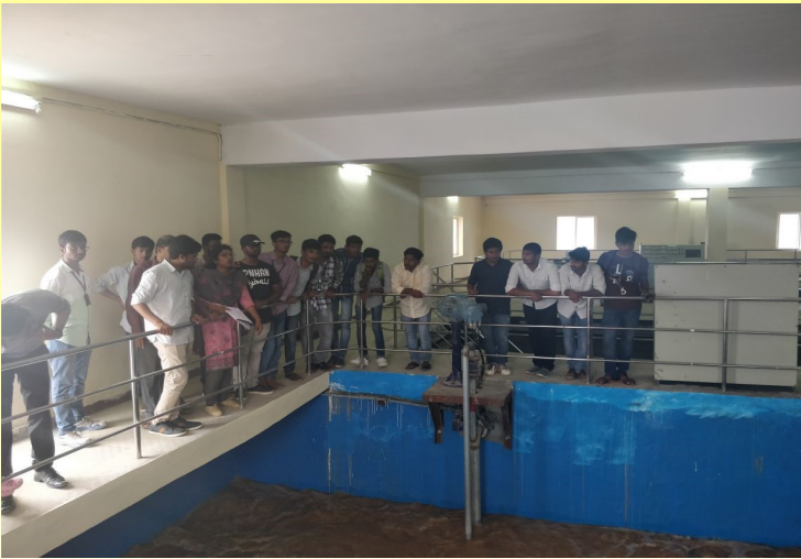
Technical Field visit to “ Water Treatment Plant ”, Kammadanam Village on 28 th July 2018
